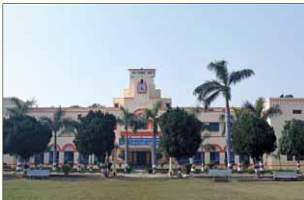
Administrative building of College of Veterinary Science
