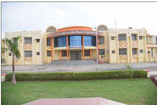
University Administrative building
