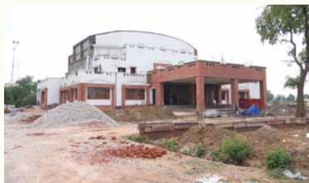
Under construction University Auditorium
