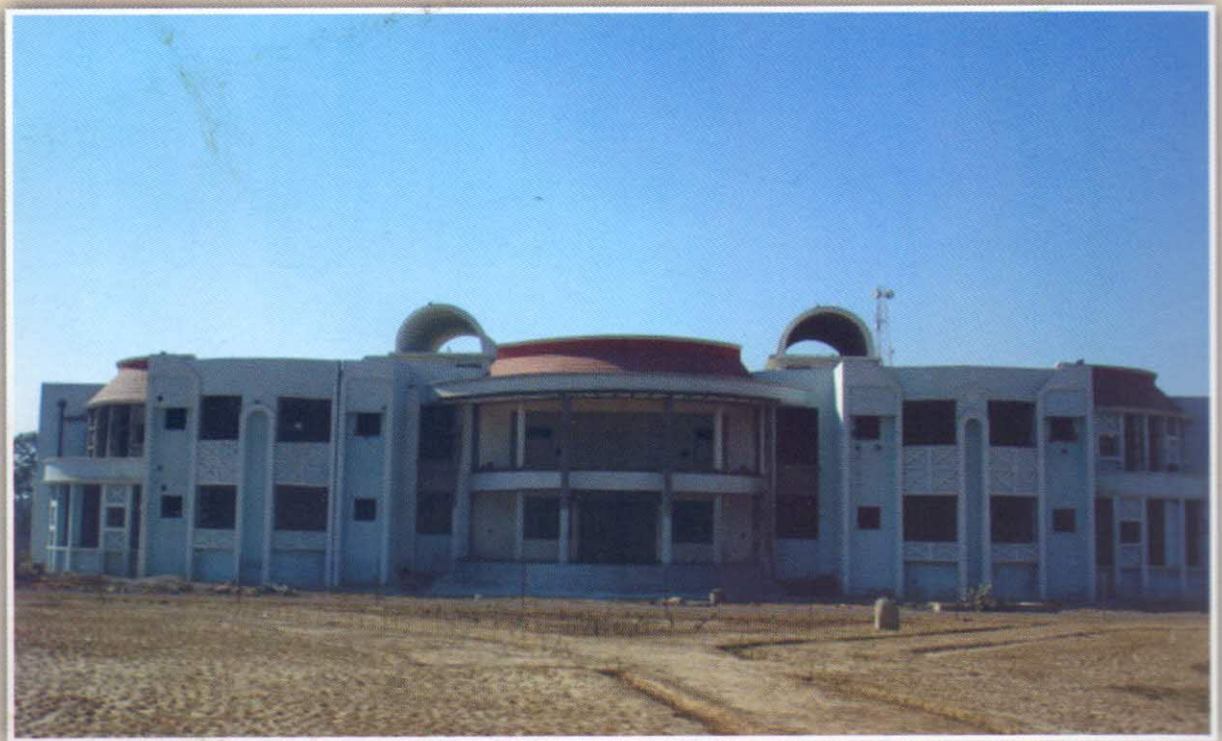
NEW ADMINISTRATIVE BLOCK
